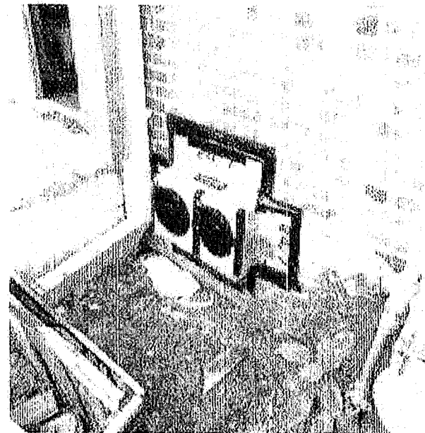
Crawl Space Vent fan.
